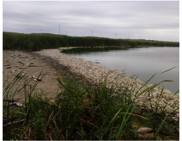
Headwater lake for Twin renovation 2015
