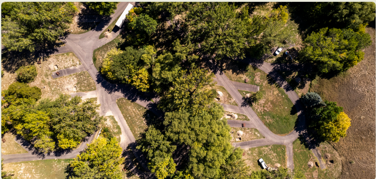
A proposed project will accommodate upgrades to 50-amp service at Solider Creek Campground at Fort Robinson State Park in Dawes and Sioux counties. JUSTIN HAAG, NEBRASKALAND
