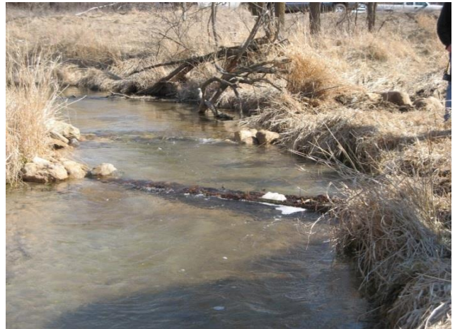
Photo 24: Spur log structure
