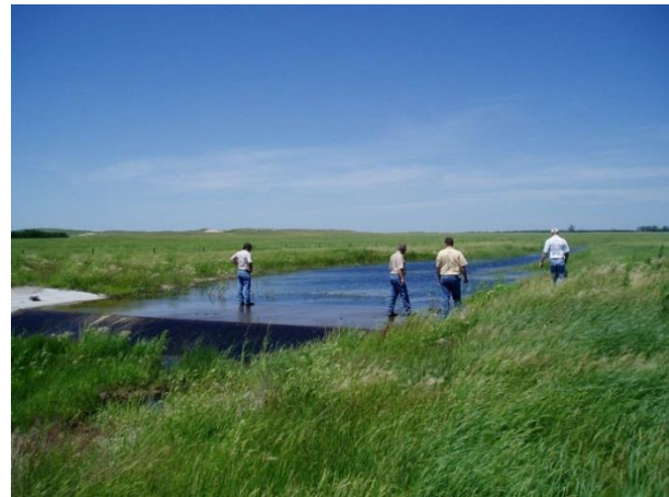
Photo 18: Water control structure
