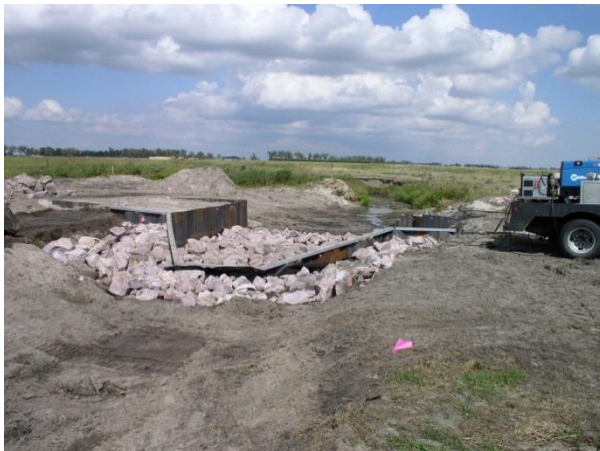
Photo 17: Weir structure on Sandhills stream
