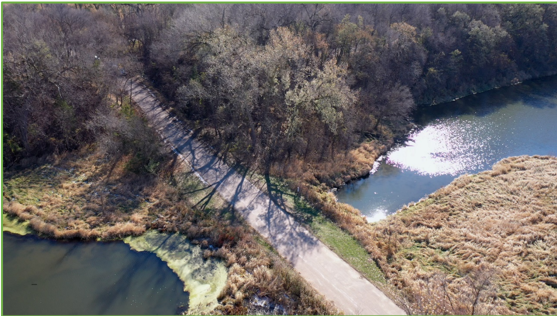
East Bridge Area aerial view facing southeast, 2020
