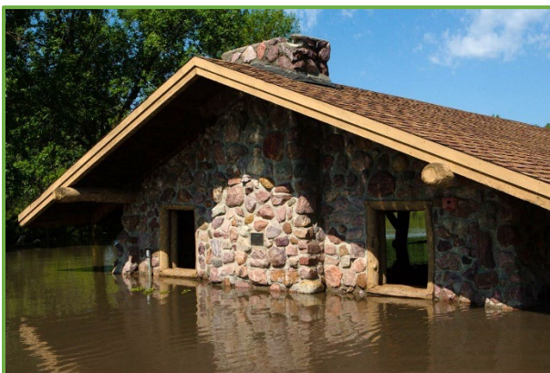
Flooded Stone Shelter House, 2010, Nebraskaland magazine
