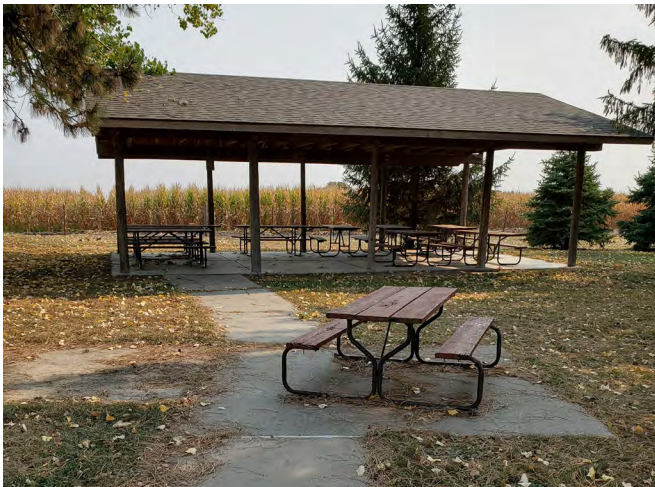
Picnic shelter and benches.
