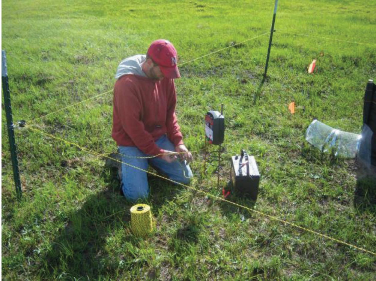
Fig. 3. Photograph demonstrates the construction of electric fences around trapping arrays to prevent disturbance by cattle. Electric fences were constructed using t-posts, yellow-black polywire, blitzers (Model 12VID-5, Zareba Systems, Ellendale, MN), bailing wire, plastic and porcelain insulators, and car batteries.
