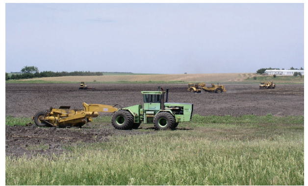
Figure 24. Sediment removal from a Rainwater Basin helps restore the full suite of wetland functions. Source: Randy Stutheit (NGPC)
