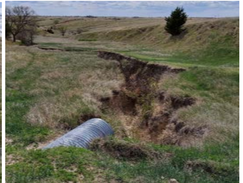
Figure 11. Gulley Erosion, Channel Incision
